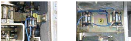
Limit switch for self-holding circuit
